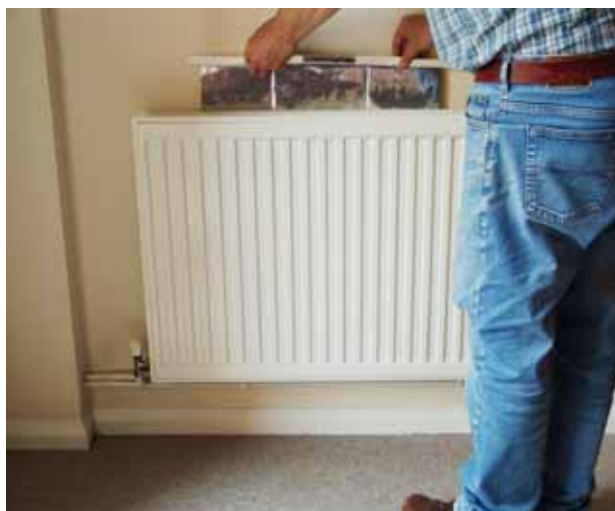
Fitting radflek behind a panel radiator
