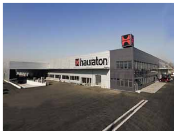
Hauraton new production and distribution facility Otigheim, Germany
