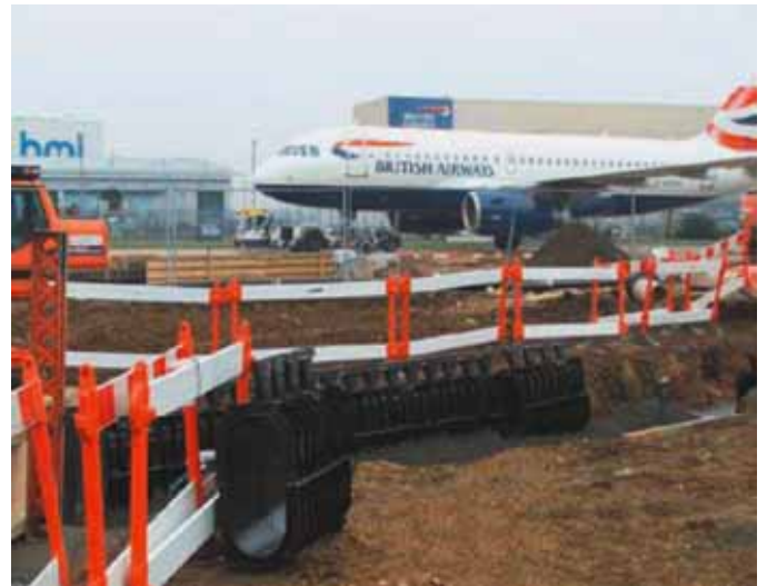
RECYFIX® HICAP® being installed at BAA Heathrow
