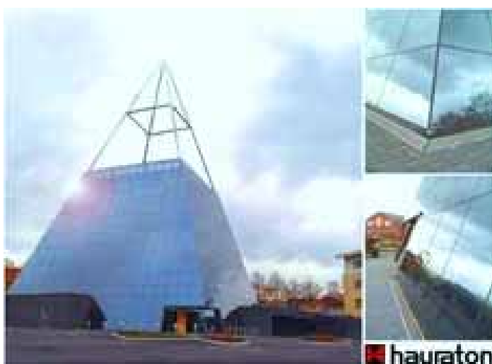
Photographs shows The Inspire building
