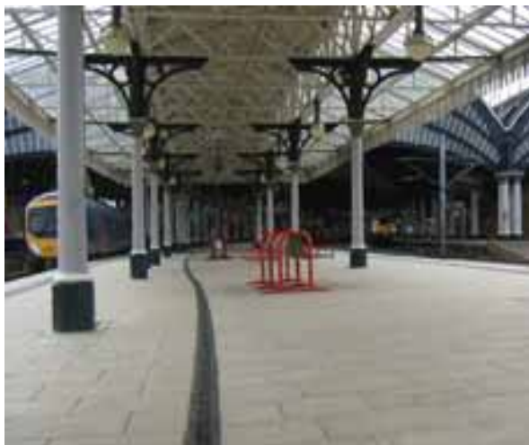
Platform surface drainage - York Rail Station
