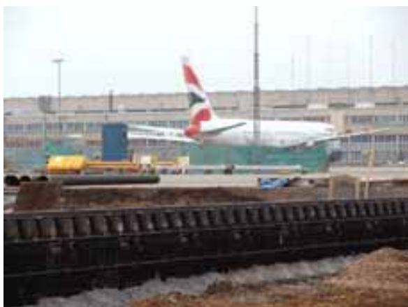
Installation of Hauraton®RECYFIX HICAP at London Heathrow
