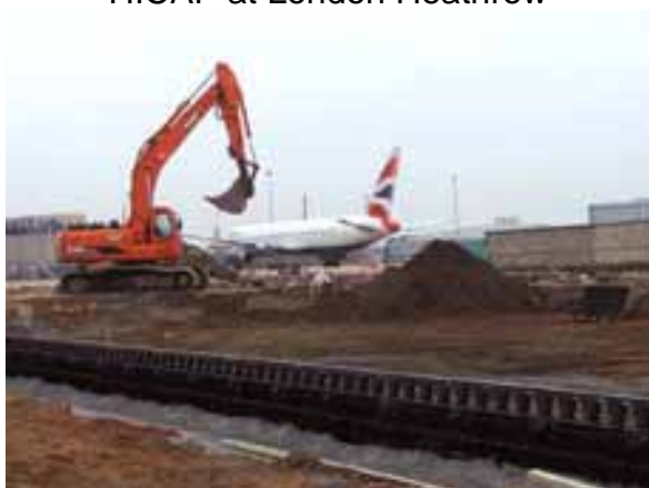
Installation of Hauraton®RECYFIX HICAP at London Heathrow
