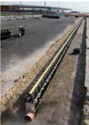
Hauraton RECYFIX® HICAP Slot drainage channel in car park
