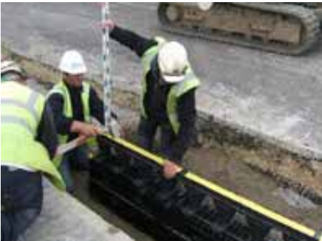
Hauraton RECYFIX® HICAP Installation of slot drainage channel
