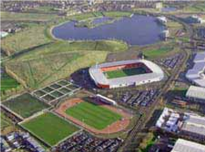
Doncaster Community Sports Complex
