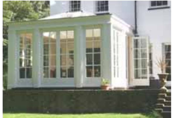
Orangery with SpanGard roof
